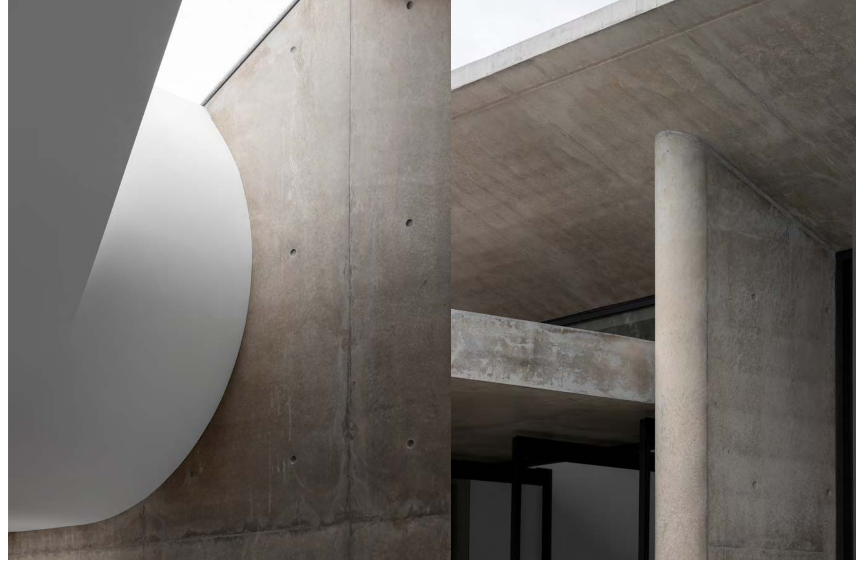
A concrete shroud sloping upwards invites sunlight into the space, providing incredible light play across surfaces.
